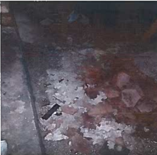
Asbestos debris mixed into dirt floor
