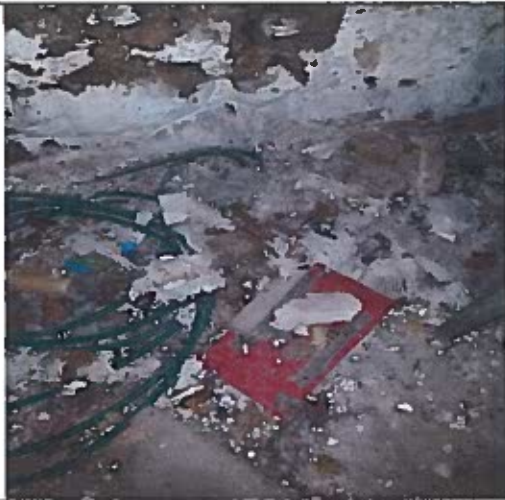
Asbestos debris in basement
