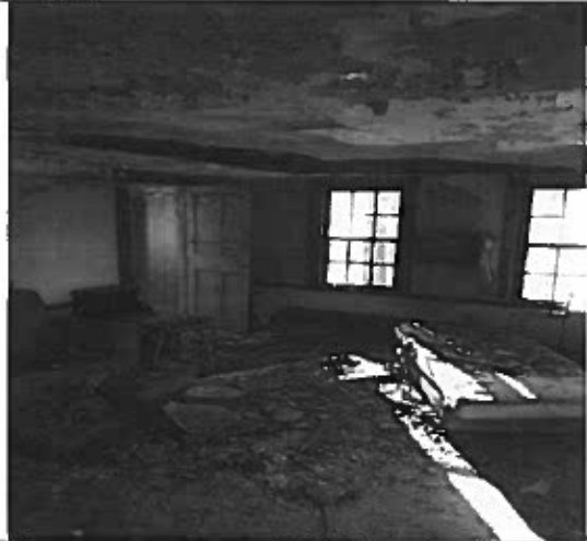
Historic house general floor 2 view
