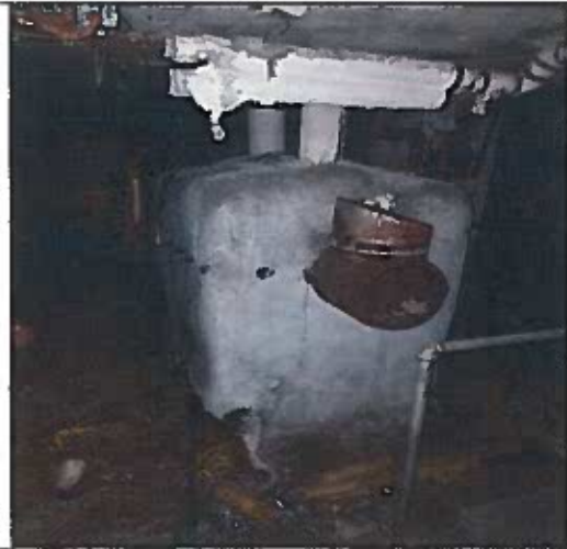
Boiler & pipe insulation
