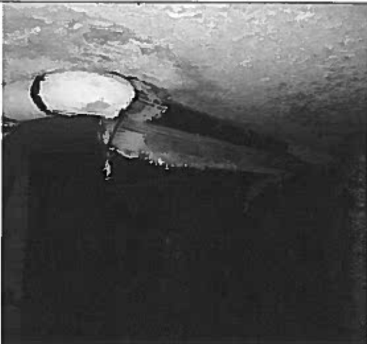
Damaged asbestos pipe in basement
