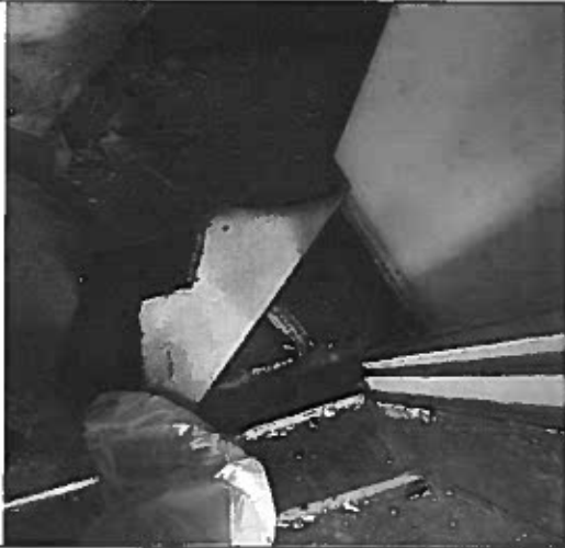
Floor tile under carpet
