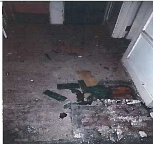
9" floor tile in floor 1 room
