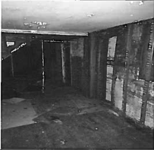
Historic house general floor 1 view
