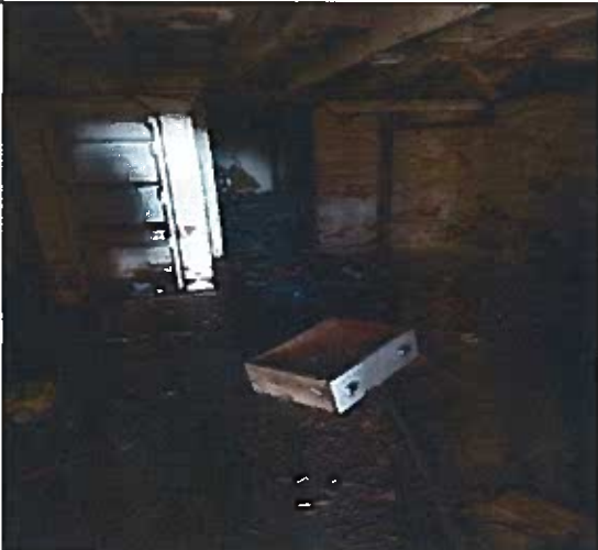
Basement section with 9" floor tile and debris
