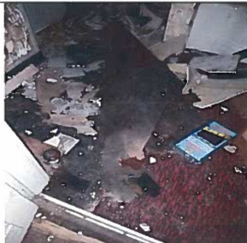
Debris with 9" floor tile under carpet
