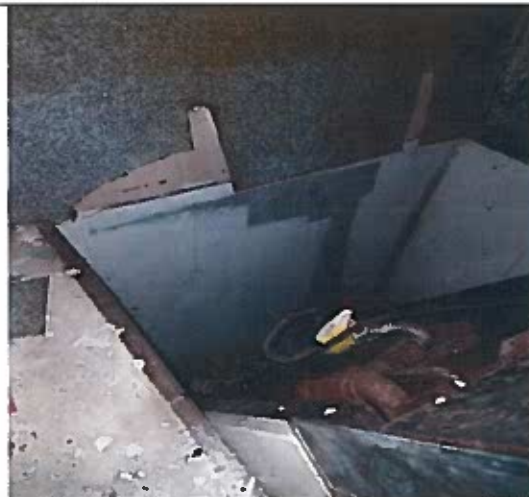
Asbestos heat board
