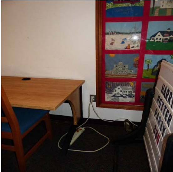
Surge protectors on the Library mezzanine
