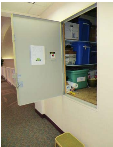
HVAC passage used as Library storage
