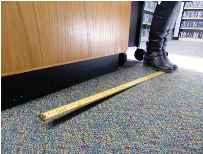
Uneven floor behind circulation desk
