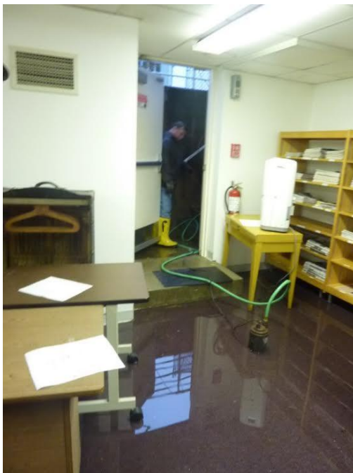
Emergency exit in basement inaccessible during flooding clean up
