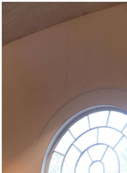
Crack above the Palladian Window
