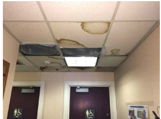
Leaking from the roof above the bathroom area
