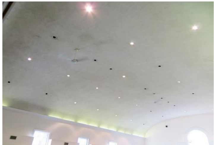
Ceiling in the main reading area and burned out bulbs
