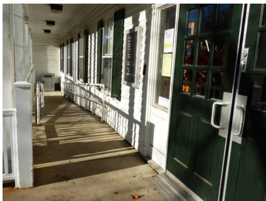
Ramp leading into Library
