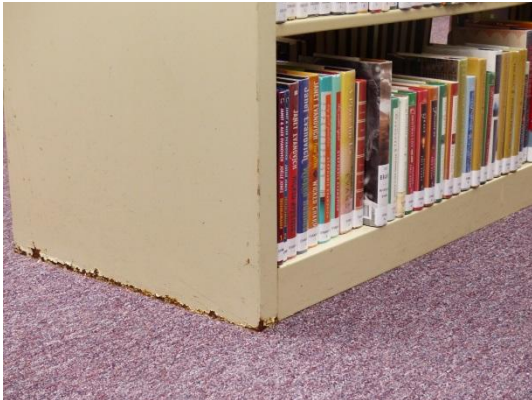
Evidence of basement flooding visible on shelving
